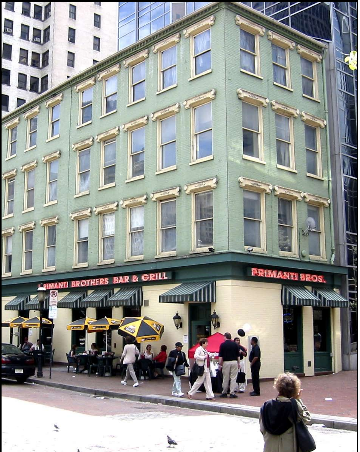
2 market square (primanti's building)
