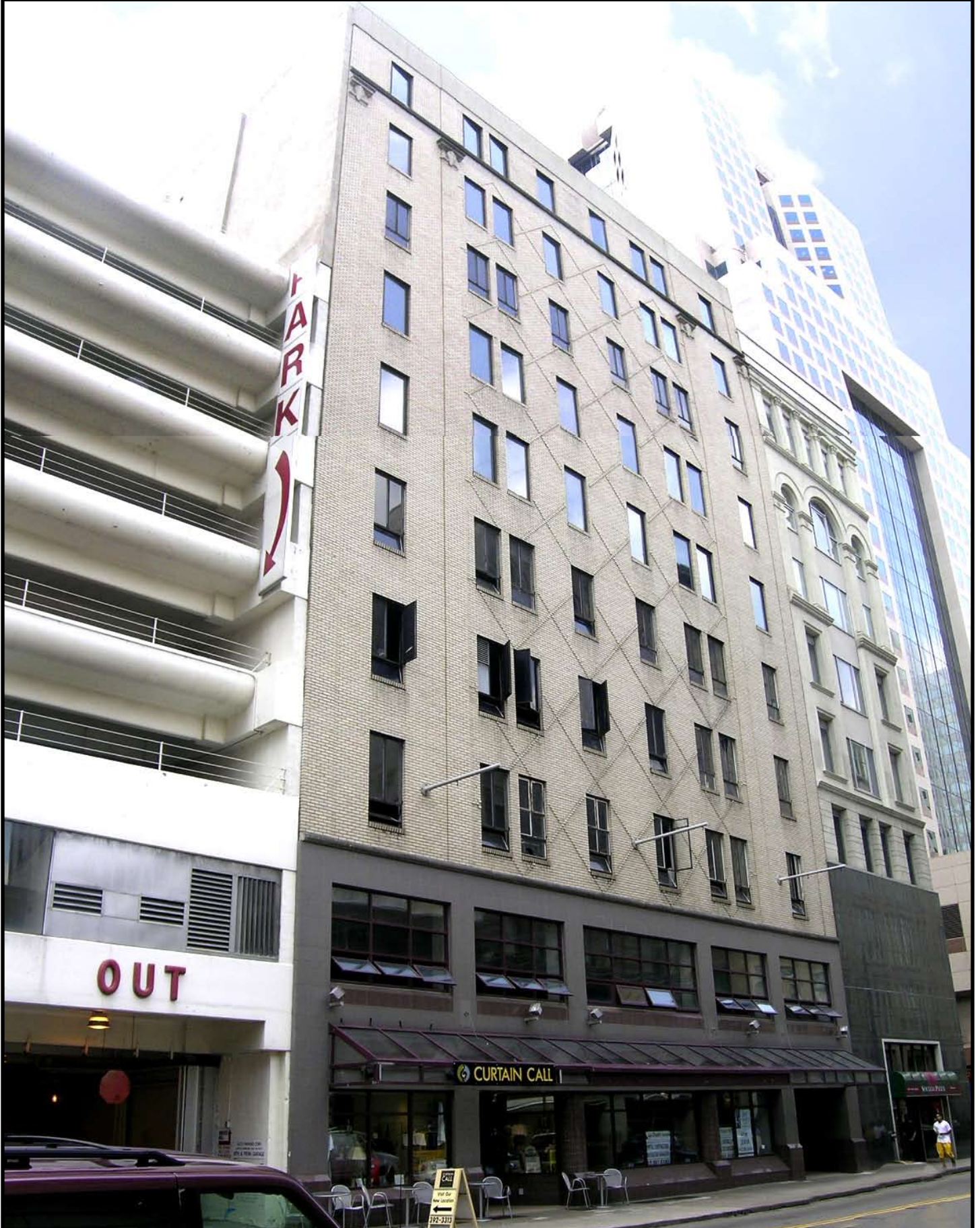
526 penn avenue (art institute building)
